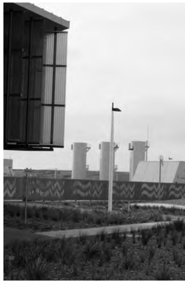
Photos by Bob Tyler of the Desalination Plant, Wonthaggi.
